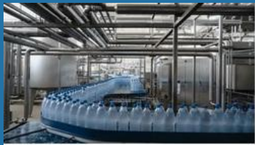
Water Bottel Plant
